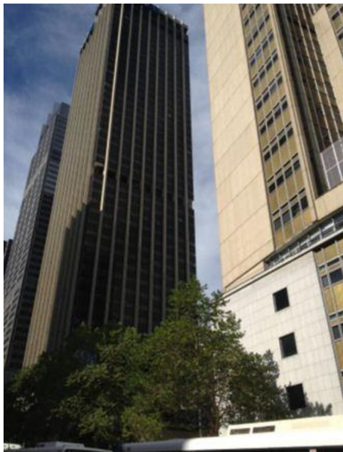
Figure 3: Site – 50 Bridge Street Tower (AMP Centre)
