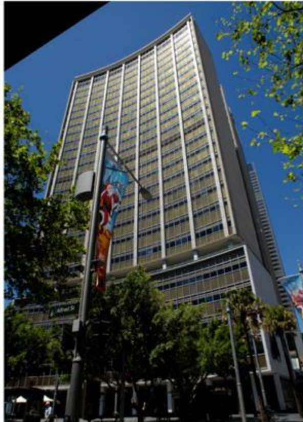
Figure 2: Site – 33 Alfred Street AMP Tower
